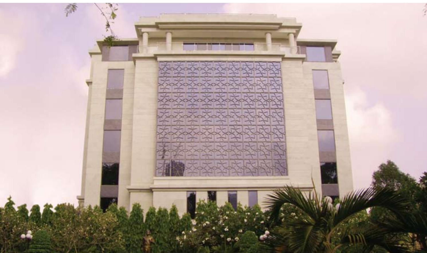
HTMC - SAVICO office building at 91 Pasteur, dist.1, HCM city
