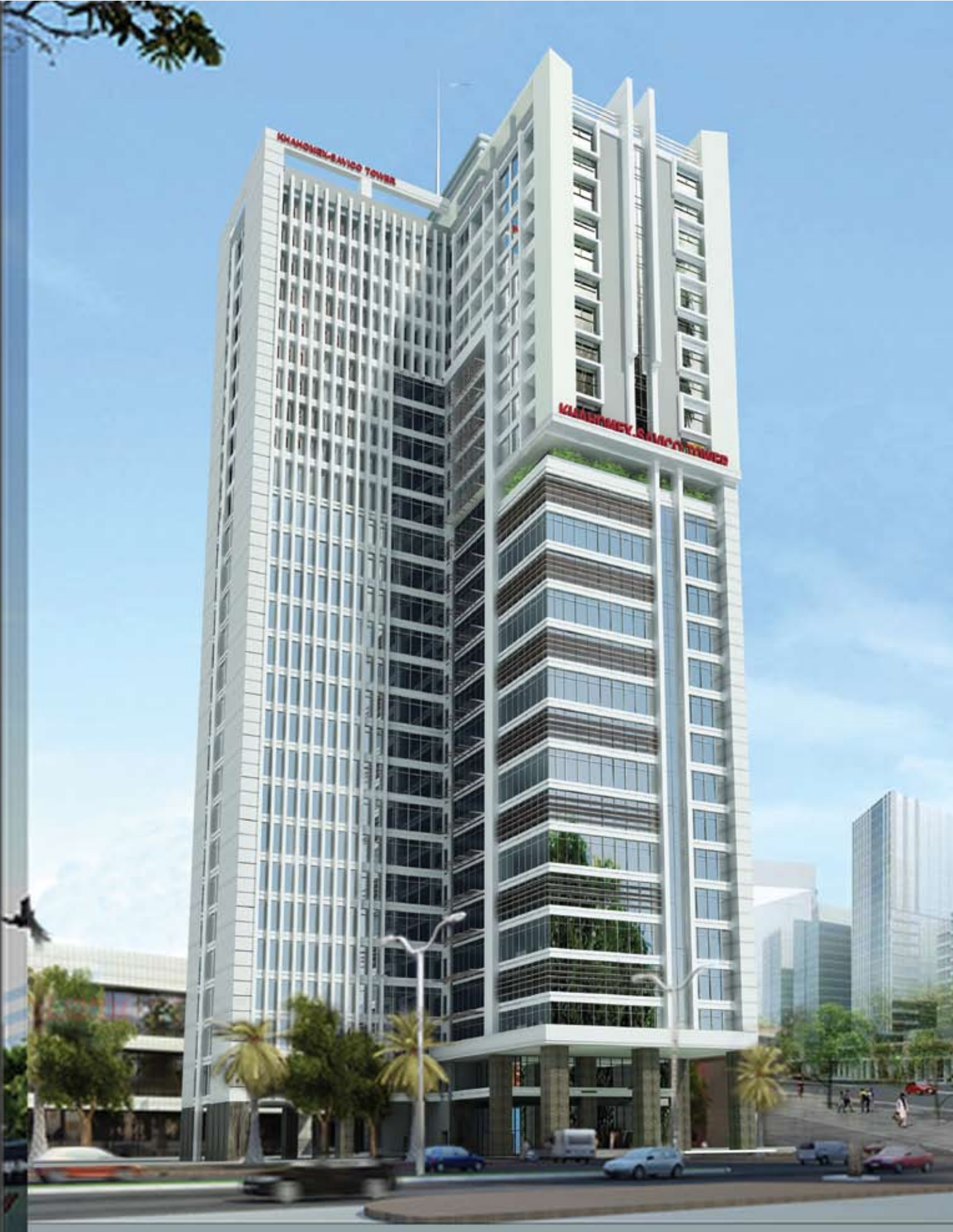
KHAHOMEX - SAVICO office building at 56 Ben Van Don, dist.4, HCM city
